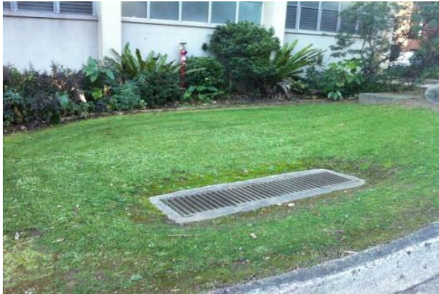
Photo 5.2.2 – Stormwater pit
