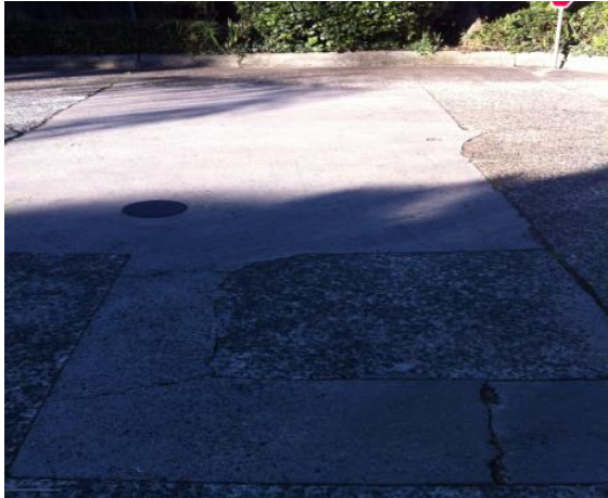
Photo 5.5.4 – Evidence of a decommissioned UST pit
