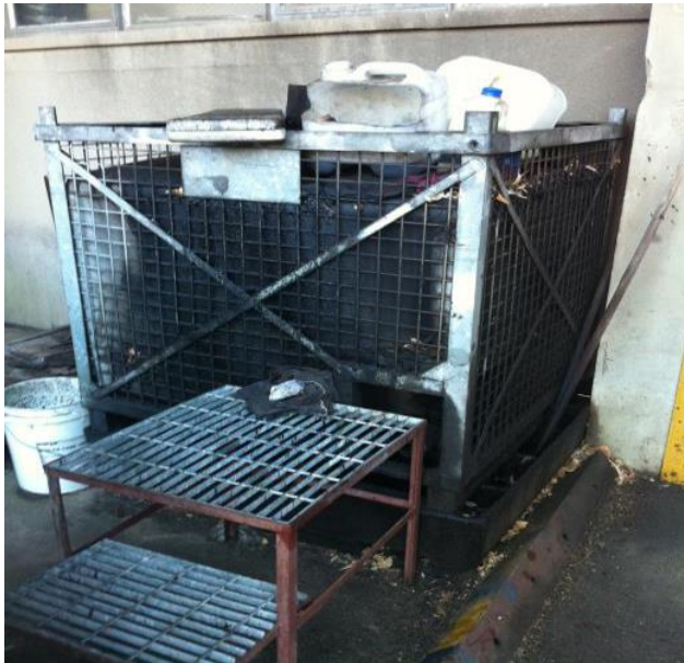
Photo 5.9.1 – Black oily substance observed to have been leaked from a mechanical equipment
