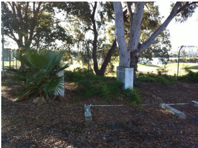
Photo 5.5.5 – Footings for former ASTs on site
